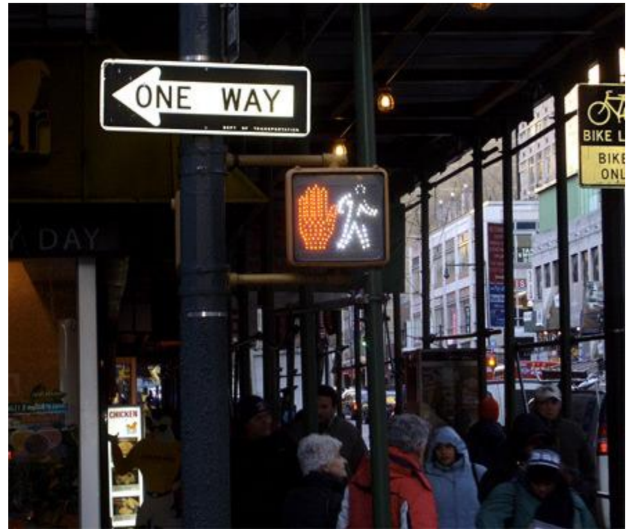
Malfunctioning crosswalk light, New York City. [Photo by Paul Hollenback ]
